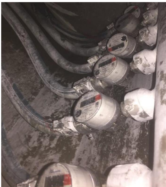
Illus. 2: flow meter units mounted in a filter tower
